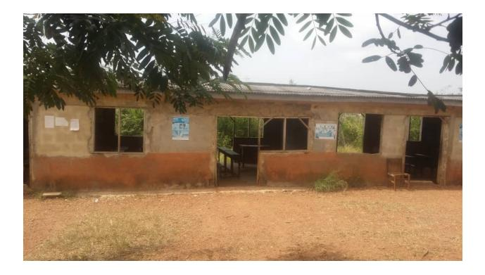
The classroom block (B) Above happens to be the Primary block of the Ekumfi, Atwea school, Which comprises of 3 three classrooms within this block. The floor of the entire block is below ground level, as the foundation of the block was not raised to the standard foundation level of our building code specifications. This may cause Sand/debris within the classrooms, and also create floods within the classrooms
