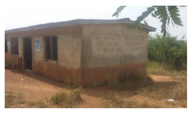
Window frames of the existing structure upon our assessment needs to be replaced due to its weak state.
